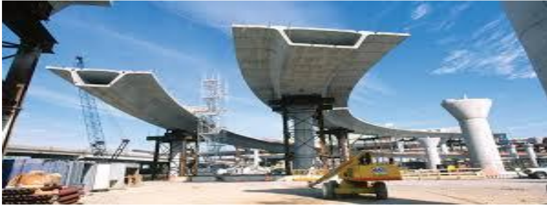
Fig-1.01: Box girder bridge for vehicular traffic movement
