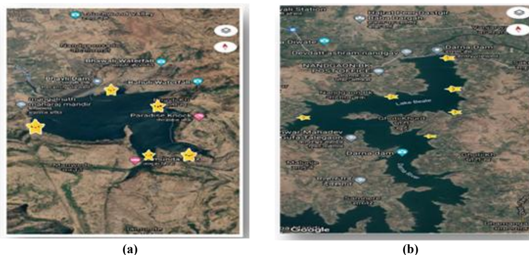
Figure: a) Bhavali dam, b) Darna dam
