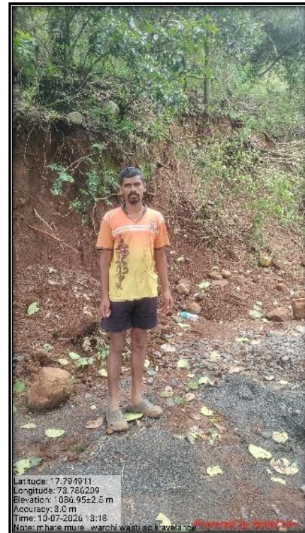
Photograph No.10 Picture showing Linear Road cutting
