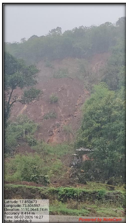
Photograph No.12 Picture showing Debris flow
