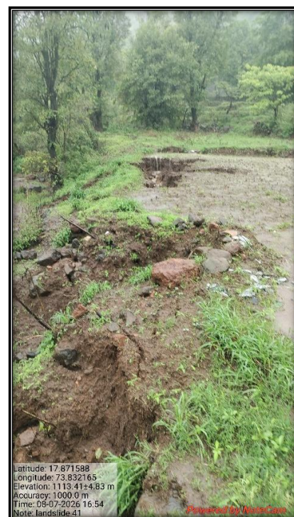
Photograph No.13 Picture showing Soil erosion
