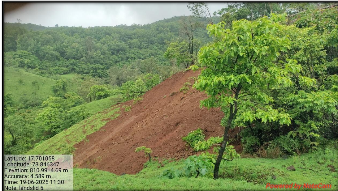
Photograph No.2 View of Landslide in Kulkajai Village
