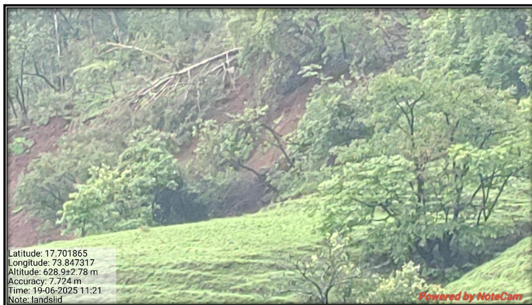
Photograph No.3 effect of Landslide in Kulkajai Village
