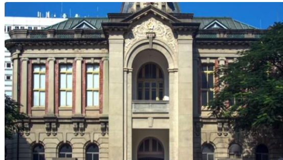
Figure 5: The exterior of the hall's wings features intricate moldings that clearly delineate two distinct stories. The second floor incorporates Japanese-style long windows set within walls divided by four massive Ionic columns.
