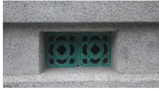
Figure 4: The parapet walls of the roof sections flanking the hall are adorned with green-glazed floral tiles commonly seen in Taiwanese residences.
