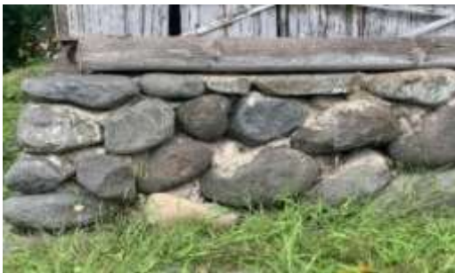
Figure: Rock foundation in the traditional house of Karang Bajo Hamlet
