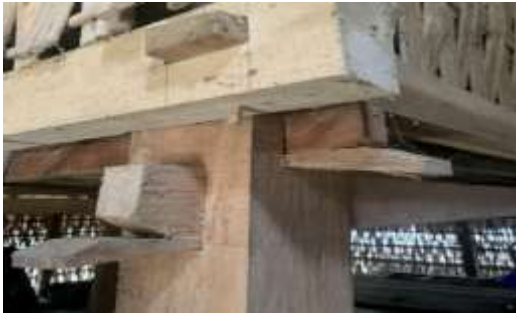
Figure: Knock down technique in traditional house of Karang Bajo Hamlet
